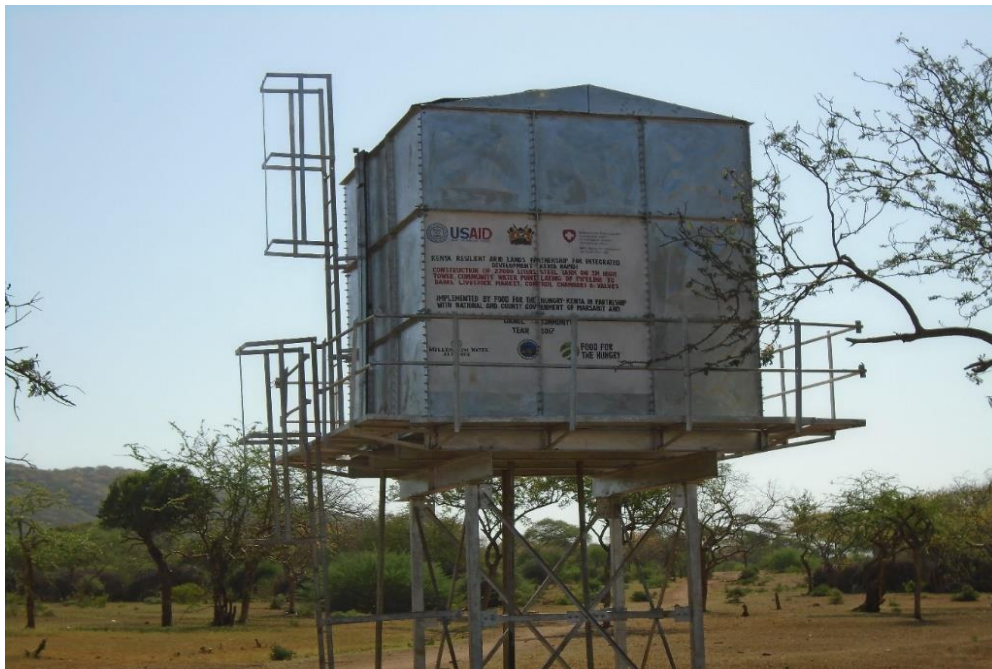
Figure 9: Water storage facility close to the project site
